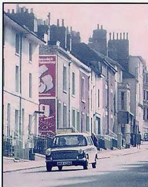
Above: Shellons Street before demolition of most of the terrace.
