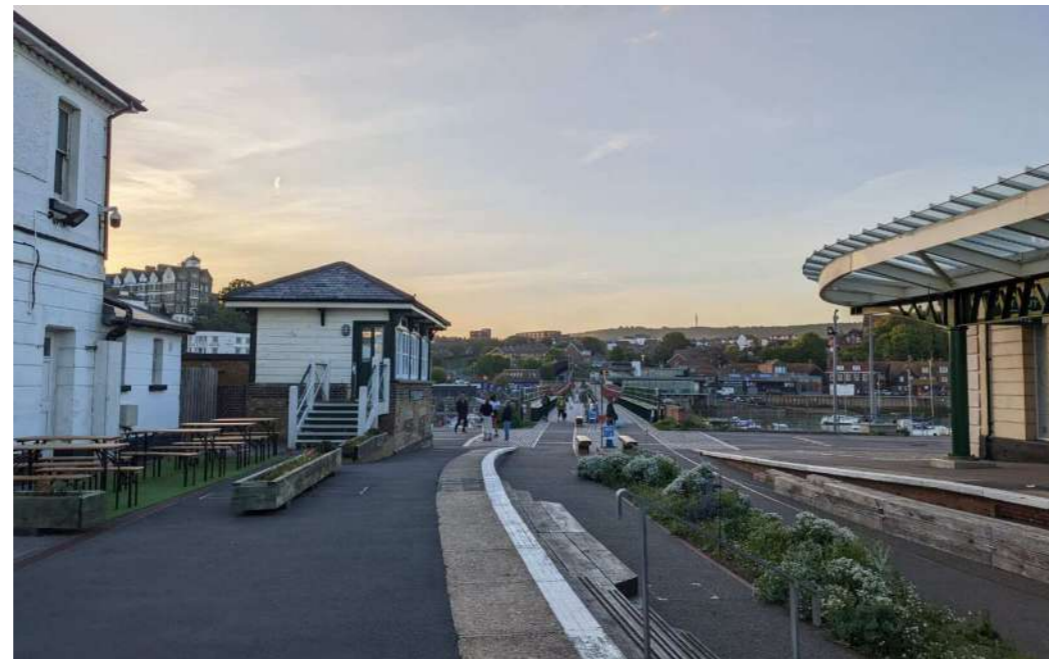
Figure 18. Harbour Station - Site photograph looking North
