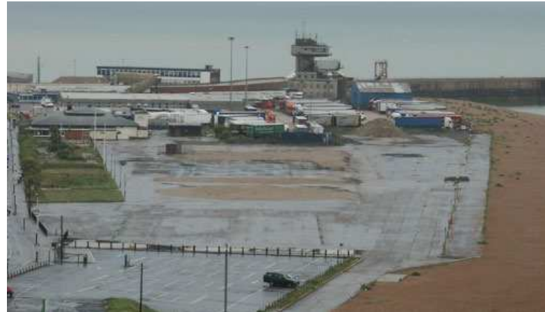
Fig 6.7.1 The Lorry Park & Concrete Beach
