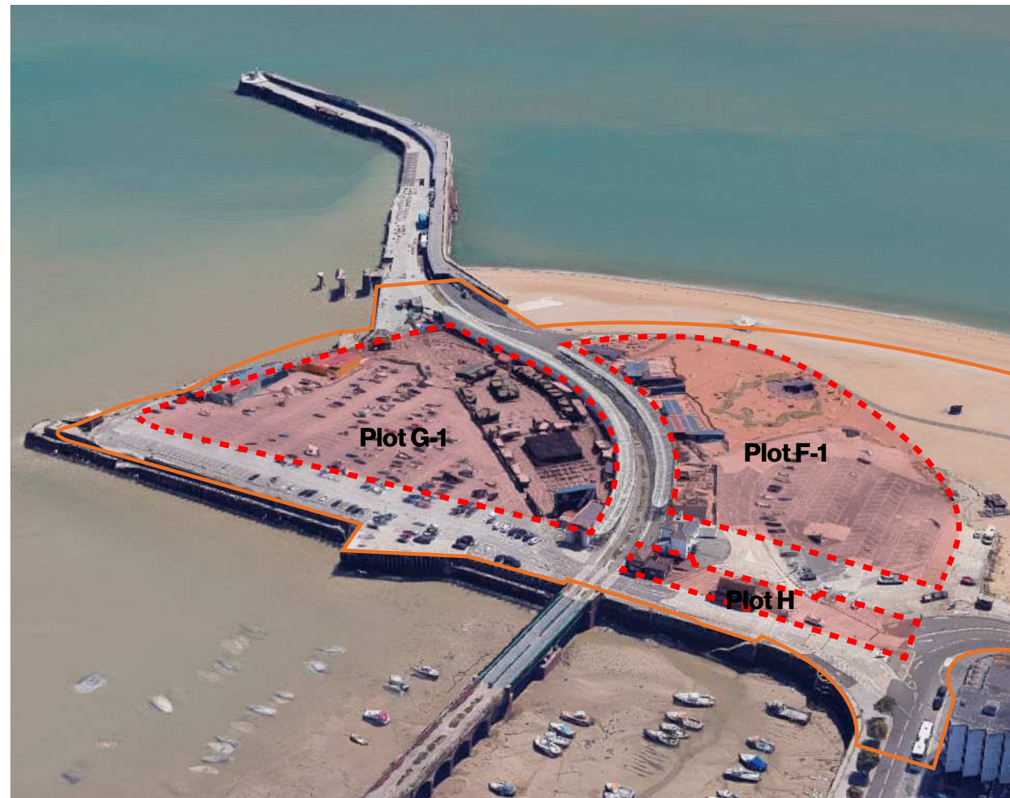
Fig 3.4.2 Plots F-1, G-1 & H aerial view north
