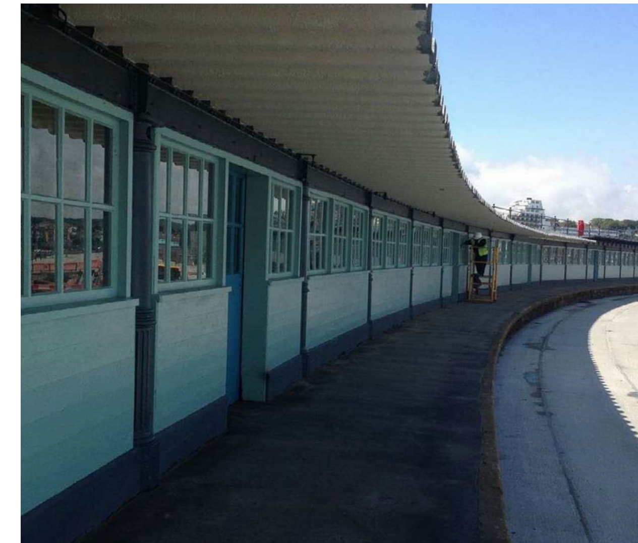
Fig 3.16.6 View of the refurbished of the waiting rooms on platform 3
