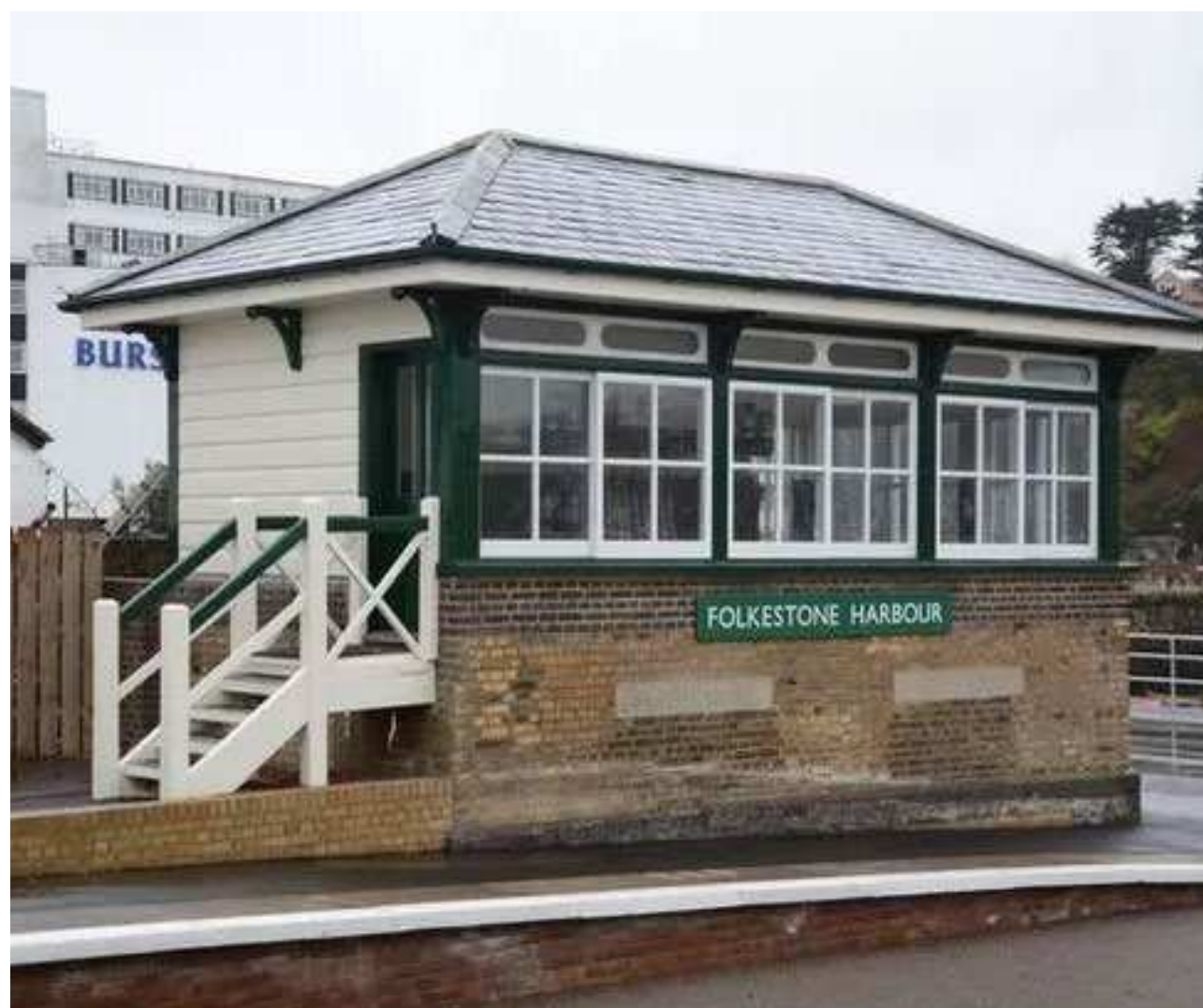
Fig 3.16.6 View of The Signal Box
