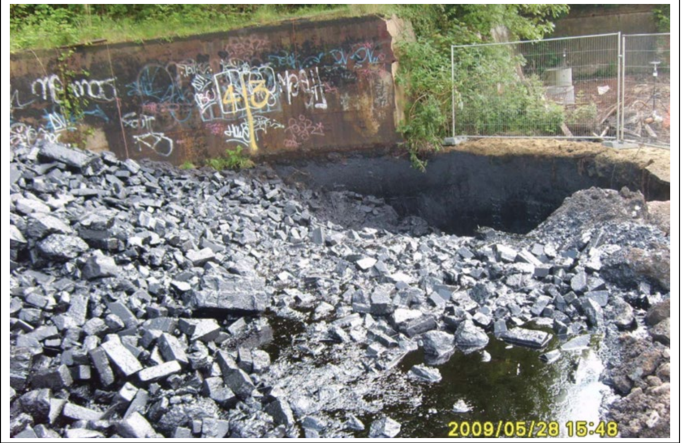
Figure 11 Excavation of contaminated material from a tank during the remediation (extracted from Mouchel Parkman factual report [8])
