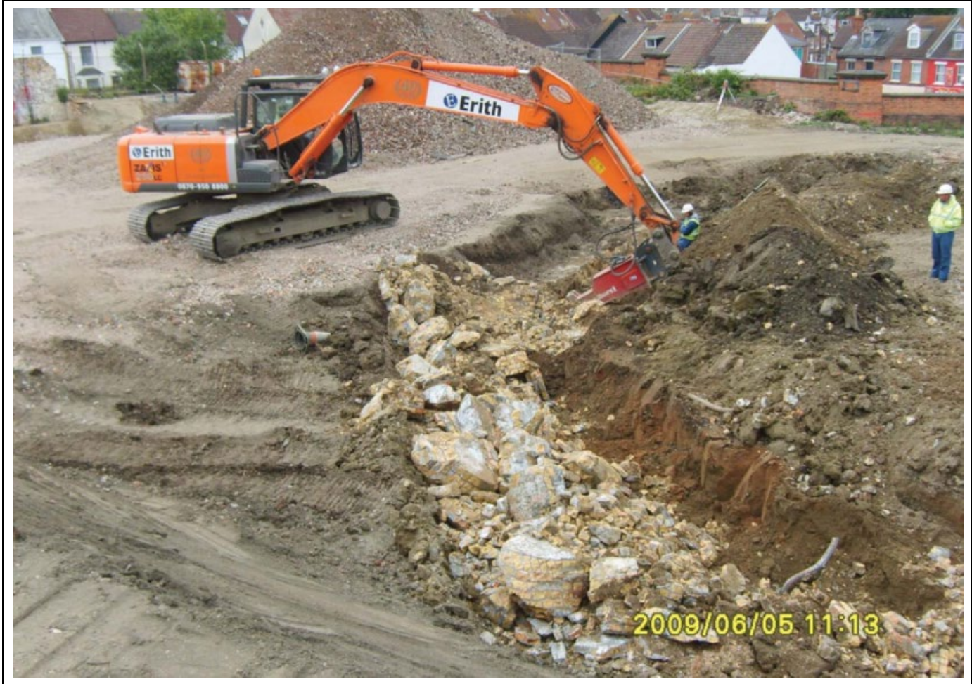
Figure 10 Partial demolition of gasholder walls (extracted from Mouchel Parkman factual report [8])
