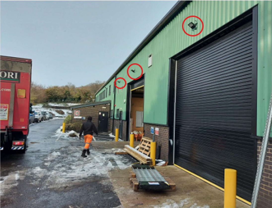
Image 4: Southern elevation – high level lights
