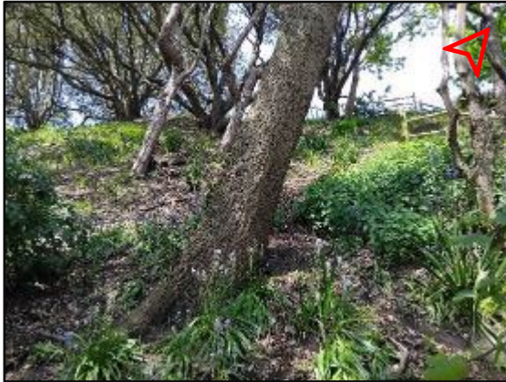
Photo 12 - Image showing the exposed soil and tree roots at L2
