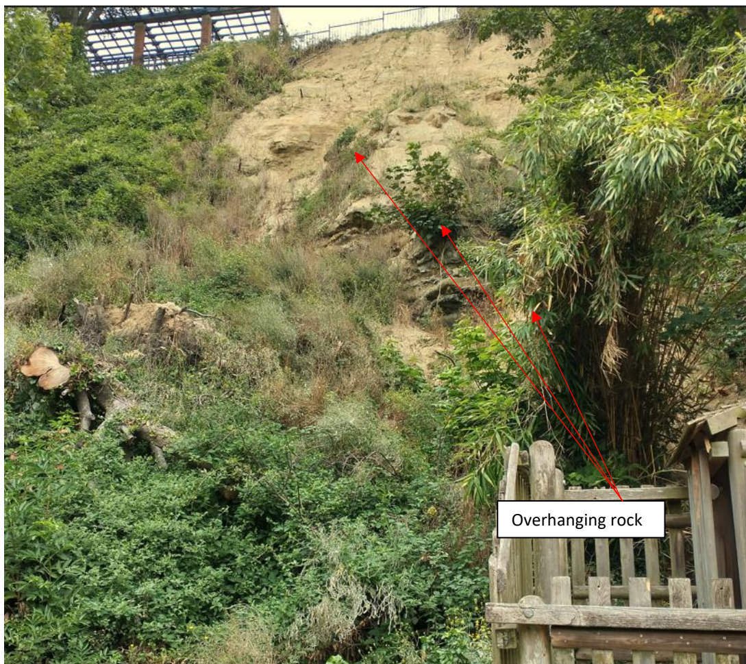
Photo 3. Photograph showing landslip, taken from toe of the slope
