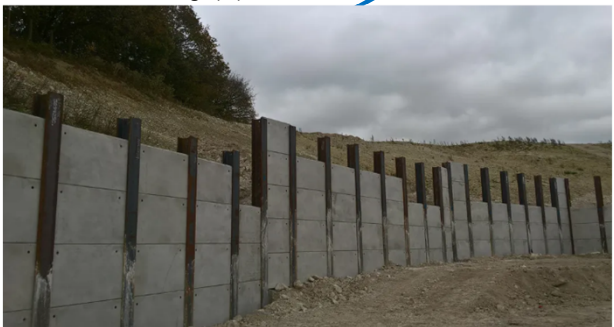
Large size king-post wall (Image belongs to Phi Group – A Keller Company)
