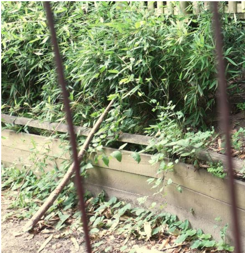
Photo 6. Timber beams form the boundary of the cliff
