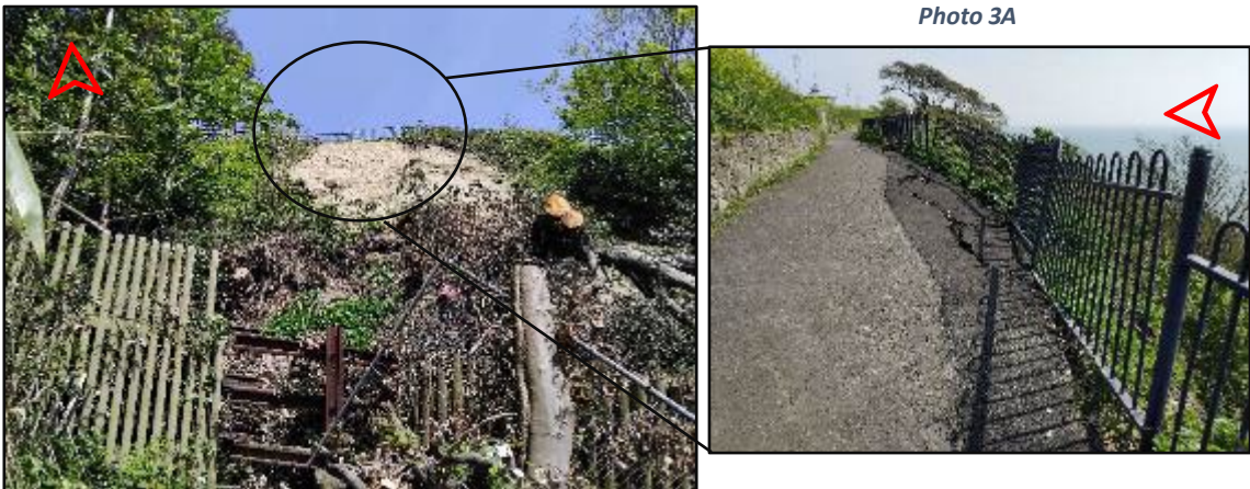
Photo 3/3A - Images taken from the northern extent of the adventure playground and at the top of the slope showing the extent of the landslide that occurred to the immediate east of 'The Vinery / The Leas Esplanade'. Photo 3A shows the continued and ongoing damage to the recently repaired asphalt path and railings.
