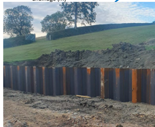
Sheet pile wall (Image taken from www.rjspiling.co.uk)
