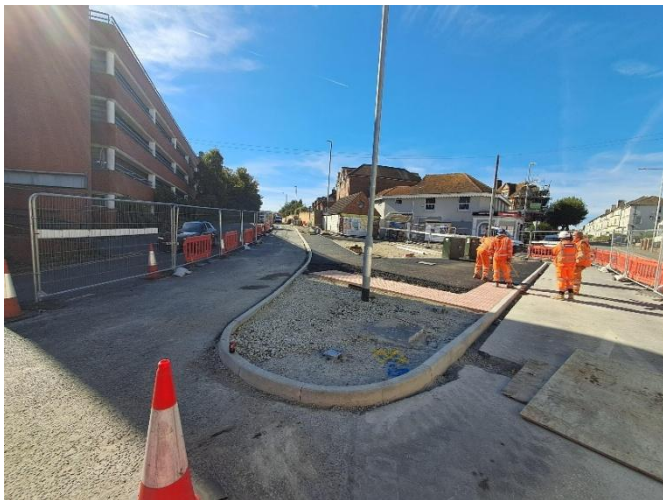
New kerbs and footways being installed along Middelburg North.
