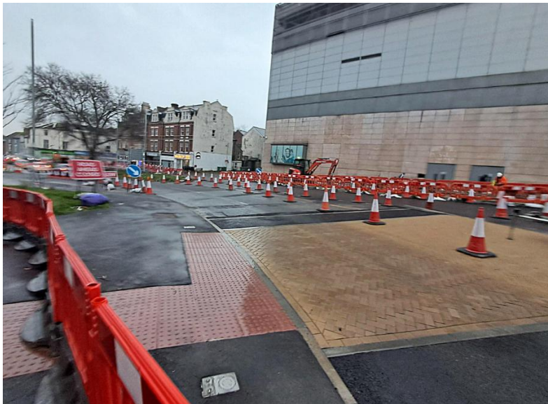
Traffic Management switched at Middelburg East – newly constructed tabletop crossing.
