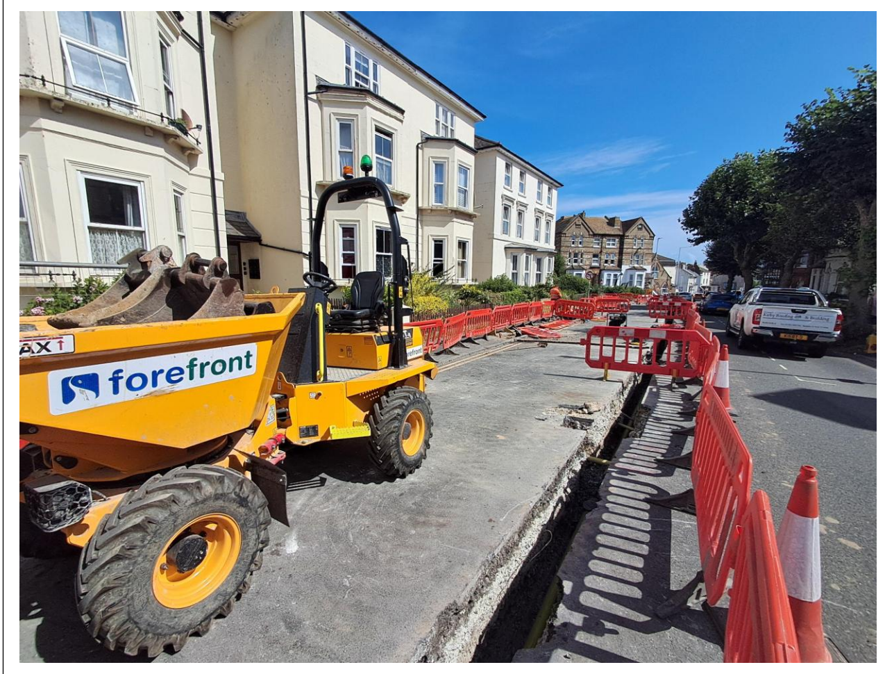
Gas diversion works located along Cheriton Road.
