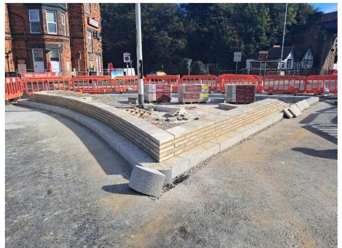
New island works at Radnor Park roundabout.
