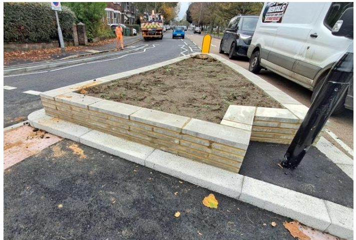
Newly constructed planters, and prepared topsoil
