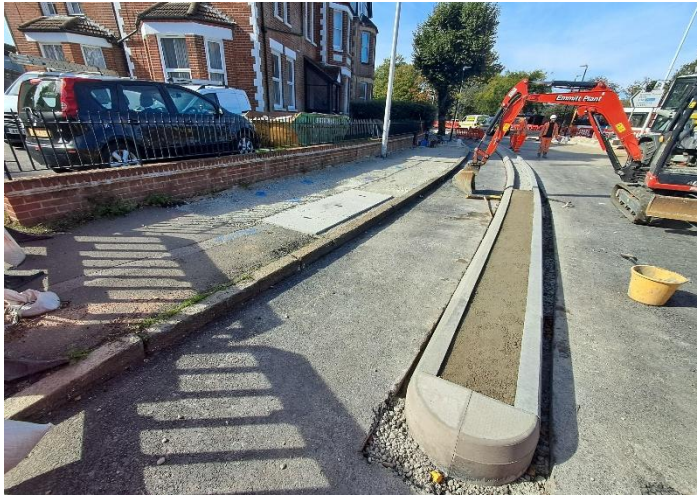
New kerbs and works for cycleways near Radnor Park roundabout.
