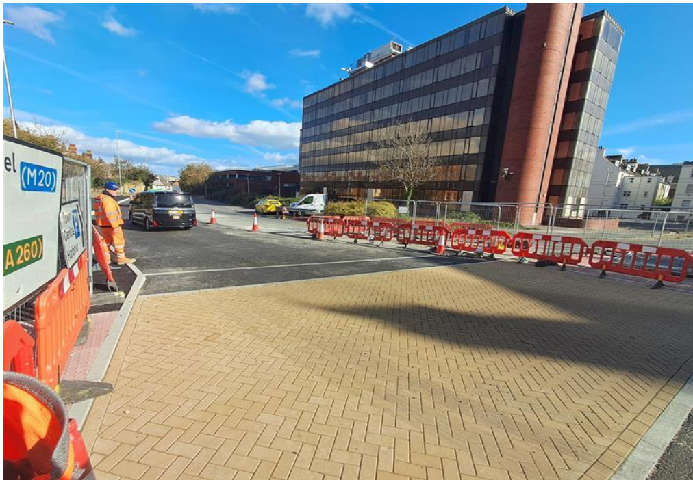
Raised tabletop crossing at Middelburg West.
