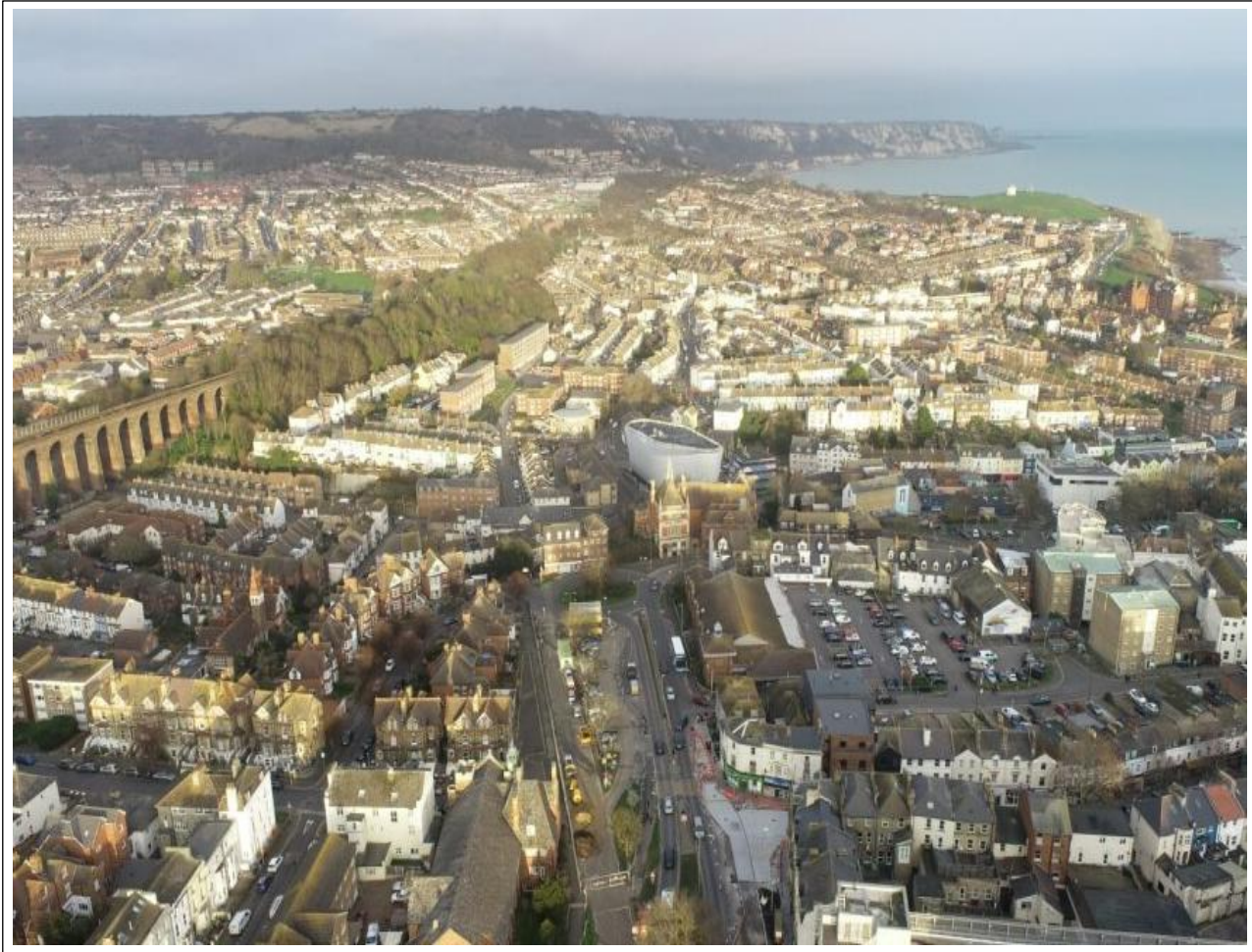
Aerial shot of the site compound and Folkestone.
