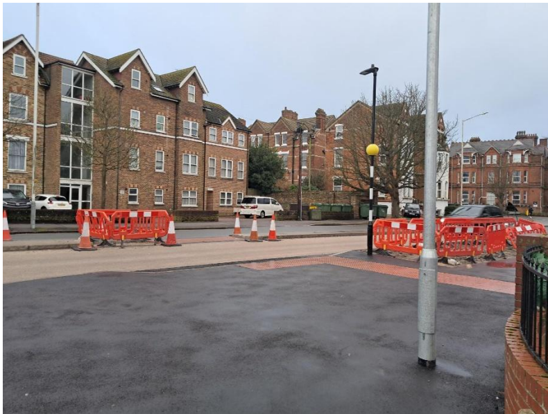
Resurfaced pavement, and Belisha Beacons at Shorncliffe junction.
