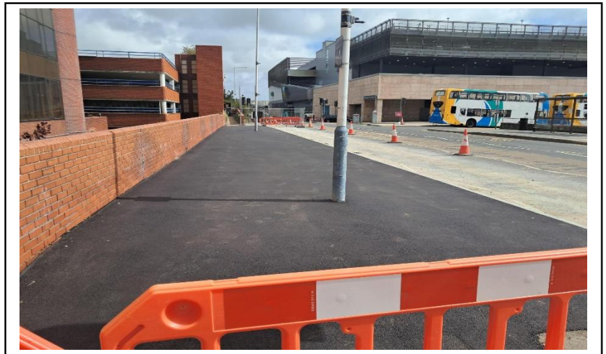
Newley resurfaced footways adjacent to the Saga building/bus station.
