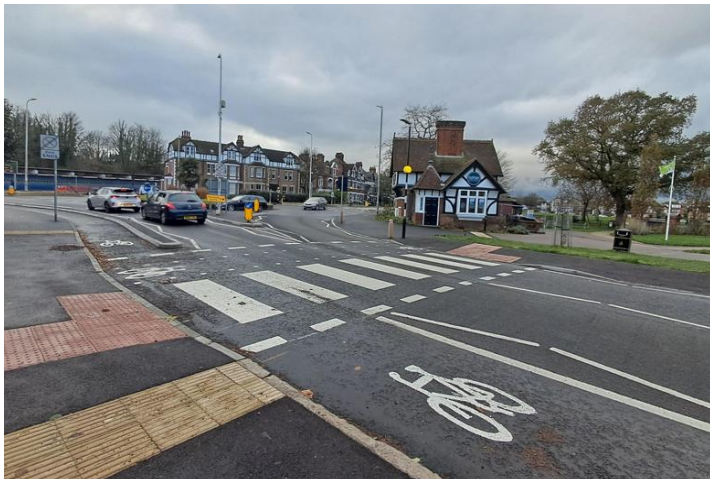
New zebra crossing, and Belisha beacons have been installed, creating safer crossing points, and cycle lanes.
