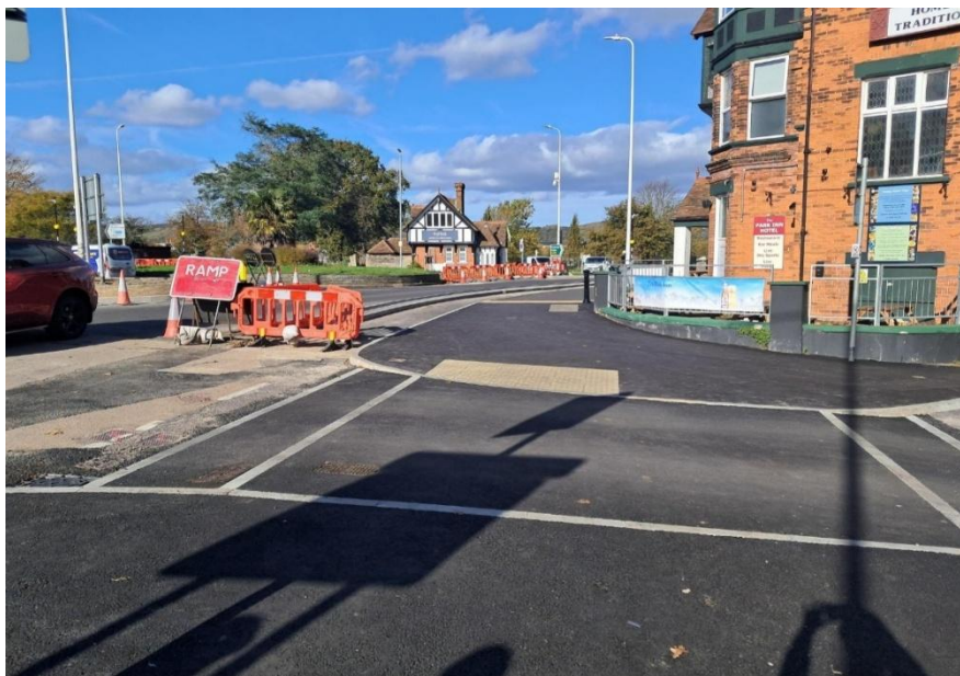
Improved junction works at Radnor Park roundabout.
