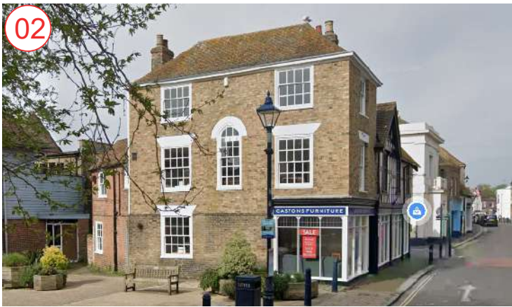
64 High Street - Grade II Listed 2.5 to 3 Storey / Buff Brick / Hipped Tiled Roof / Modillion Eaves Cornice / Sash Windows / Glazing Bars / Pseudo-timber Frame
