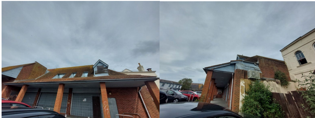
Image 01 – Buildings and hardstand dominate the site.
