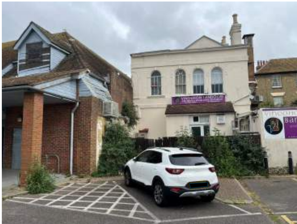
Plate 12: 74 High Street, Building of Local Merit
