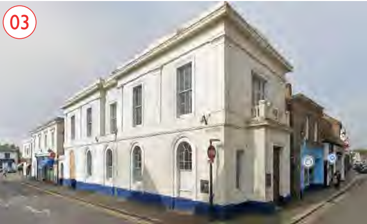
Lloyds Bank, 62 High Street 2 Storey / Stuccoed / Sash Windows / Moulded Architraves / Round Headed Ground Floor Sash Windows / Cornice Detailing
