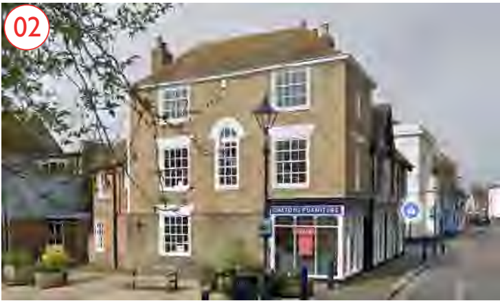
2.5 to 3 Storey / Buff Brick / Hipped Tiled Roof / Modillion Eaves Cornice / Sash Windows / Glazing Bars / Pseudo-timber Frame
