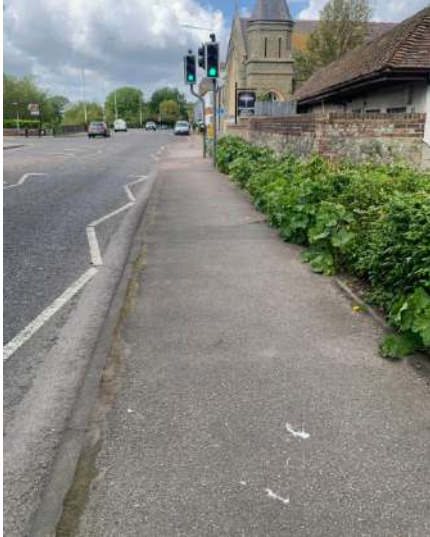
Photograph 19: A259 Footway (Northern Side)
