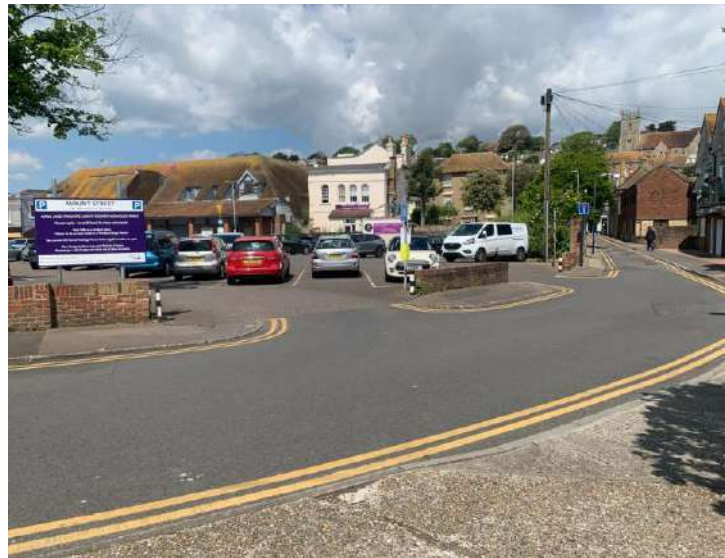
Photograph 6: Mount Street Car Park Access Arrangement
