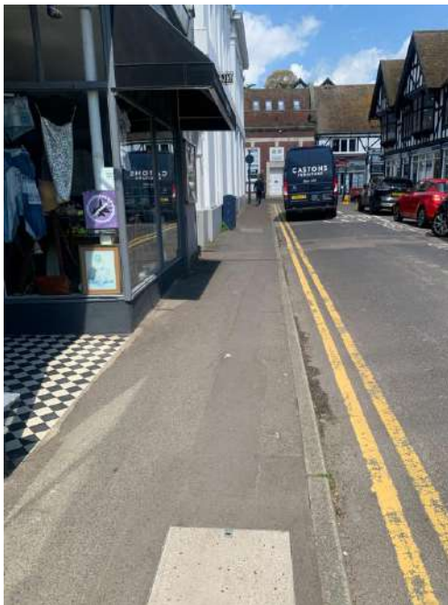
Photograph 25: Bank Street Footway (Facing North)
