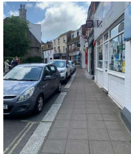
Photograph 30: High Street Footway (Facing East)
