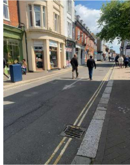
Photograph 14: High Street Existing Conditions (Facing East)
