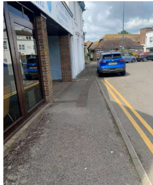
Photograph 16: Prospect Road Footway (Southern Side)
