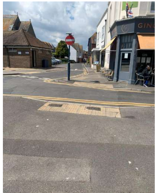
Photograph 26: Bank Street/Prospect Road Pedestrian Crossing and Chapel Street Footway
