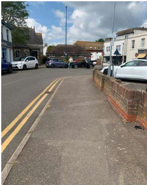
Photograph 15: Prospect Road Footway (Northern Side)
